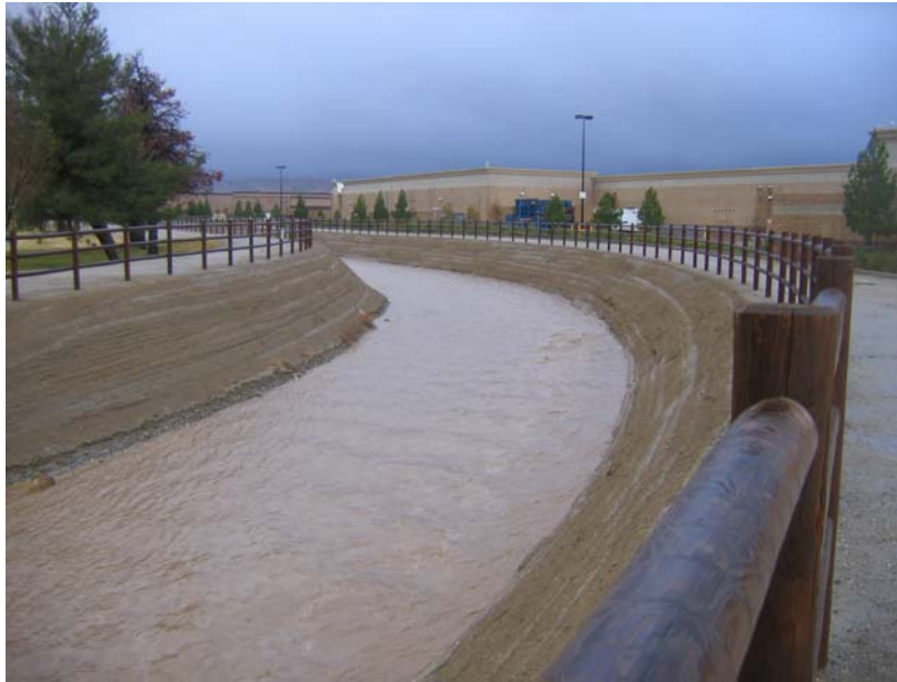
Figure 7-2: Existing Soilcrete Embankments in Amargosa Creek at Avenue O-4 (facing south)
