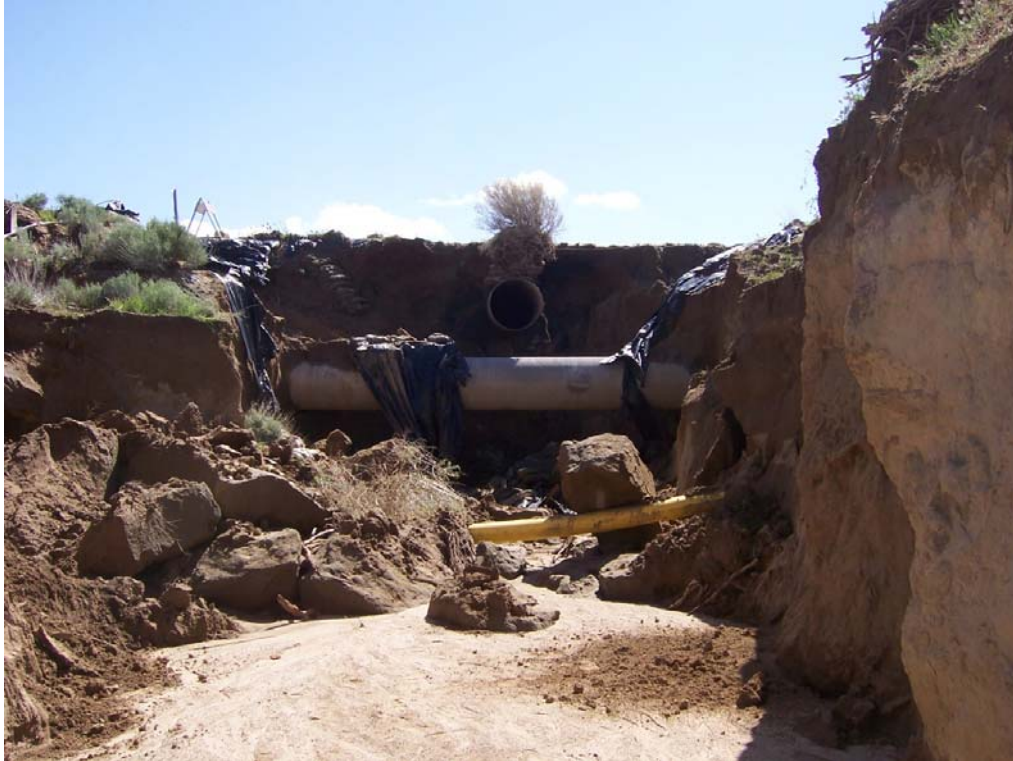
Figure 7-3: Exposed Gas and Water Pipelines from March 2011 Storm Event
